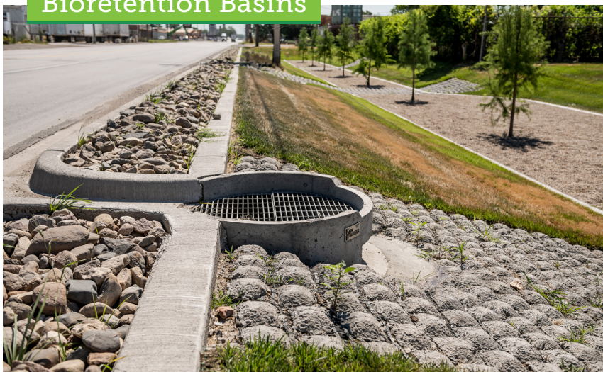
Bioretention Basins + Gravel Wetland
