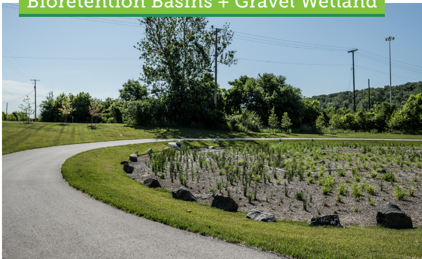
Bioretention Basins + Gravel Wetland
