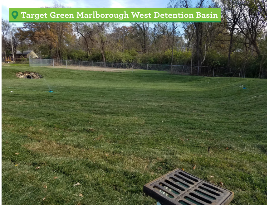
Gardner Avenue Detention Basin
